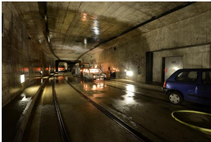
Figure 4. IFA road tunnel
